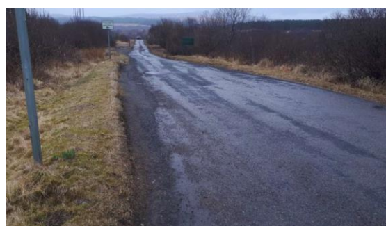
Looking south east on C47 from access to Glengorm CAS
